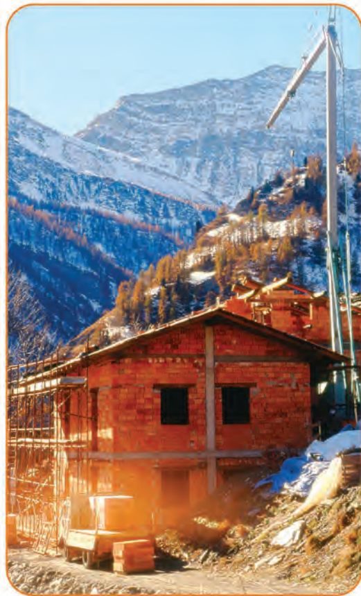
■ During the reconstruction works of the hamlet (2008-9)
